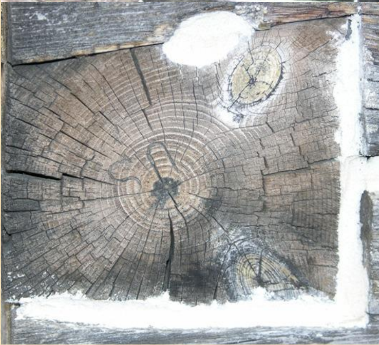
Photo 1. Log decay and animal damage to original log house. 2. "US" stamped upside down on log end.
